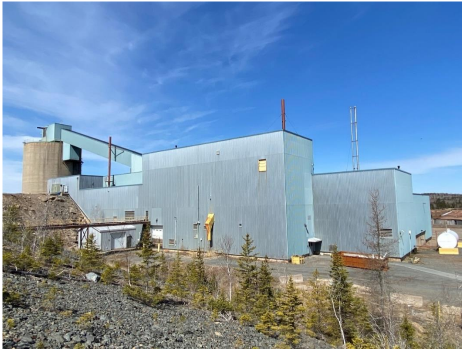
Figure 18-31: Existing Mill Processing Building – South Side Exterior View
