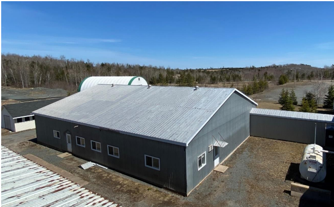
Figure 18-15: Mine Technical Services & Operations Building
