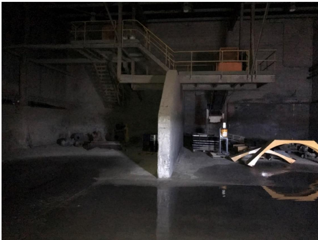
Figure 18-40: Concentrate Loadout Area
