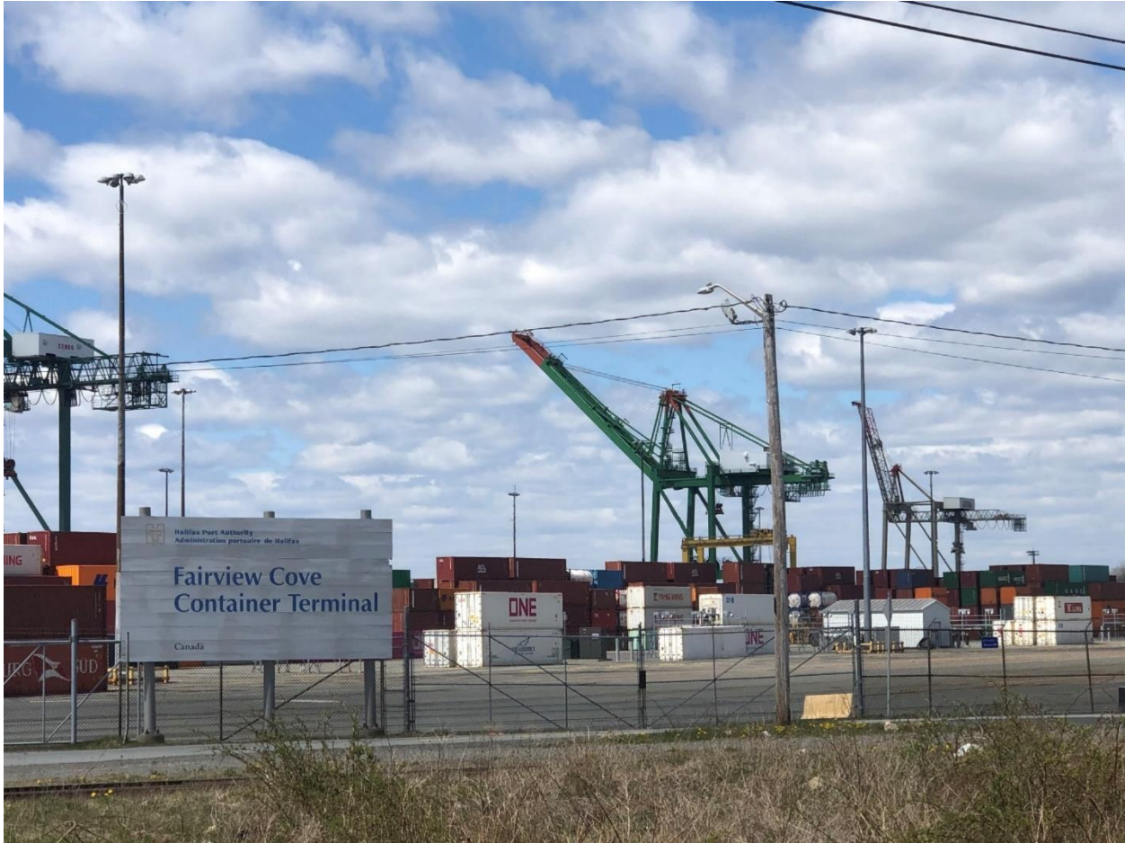
Figure 18-74: Fairview Cove Container Terminal
