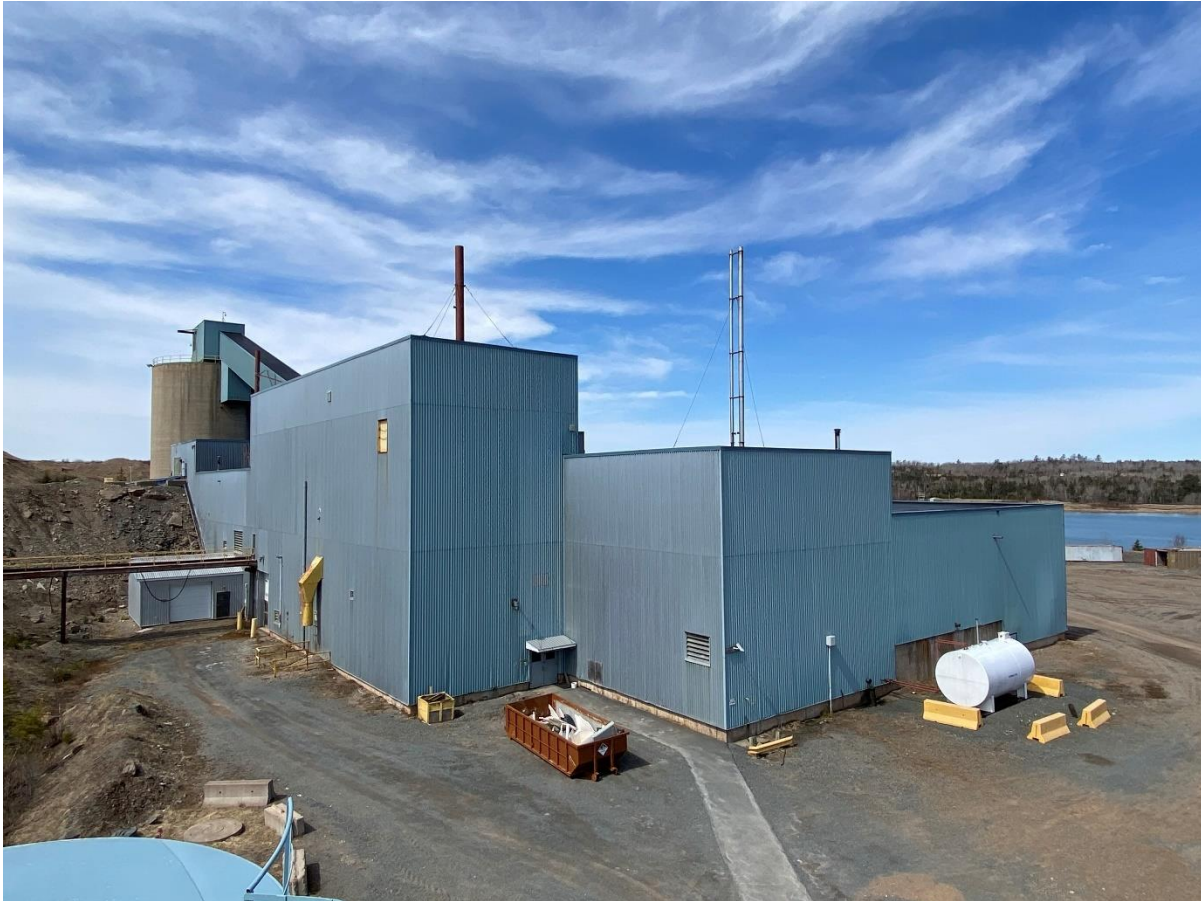
Figure 5-1: Scotia Mine Processing Facilities (or Plant)
