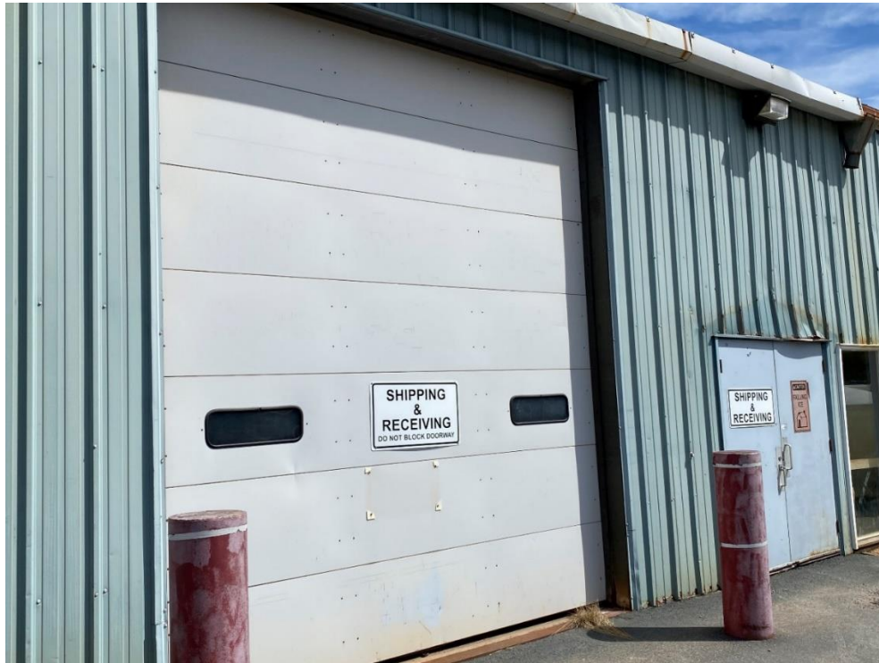
Figure 18-17: Site Warehouse Receiving Bay
