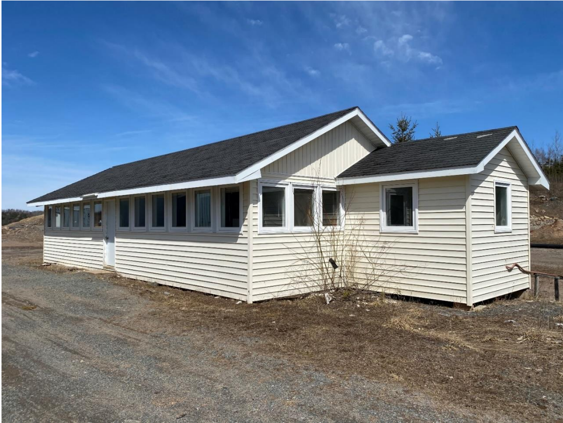
Figure 18-27: Core Preparation Building
