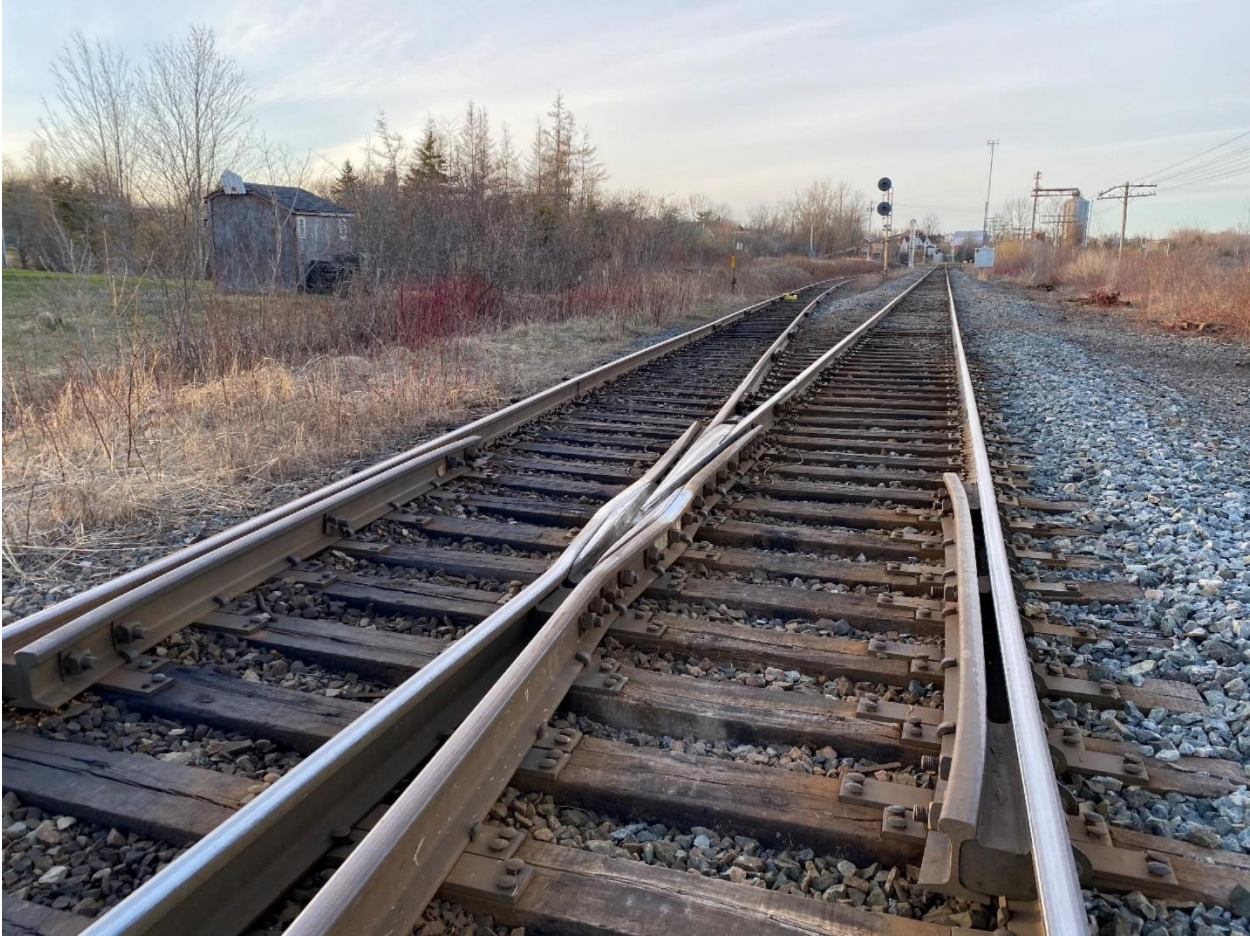
Figure 18-75: Milford CN Railway Siding
