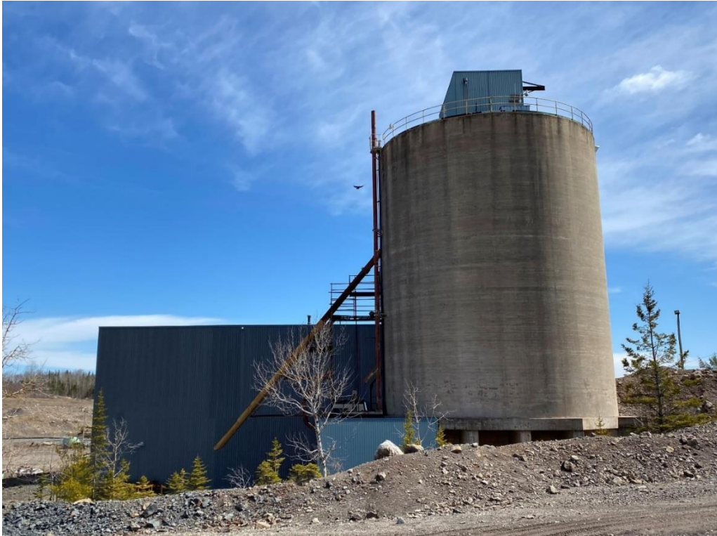
Figure 18-33: Existing Mill Fine-Ore-Bin (Silo)
