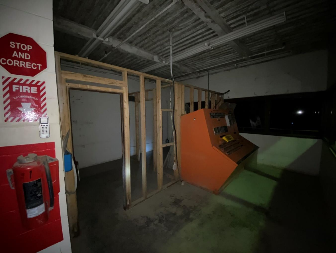
Figure 18-41: Plant Control Room
