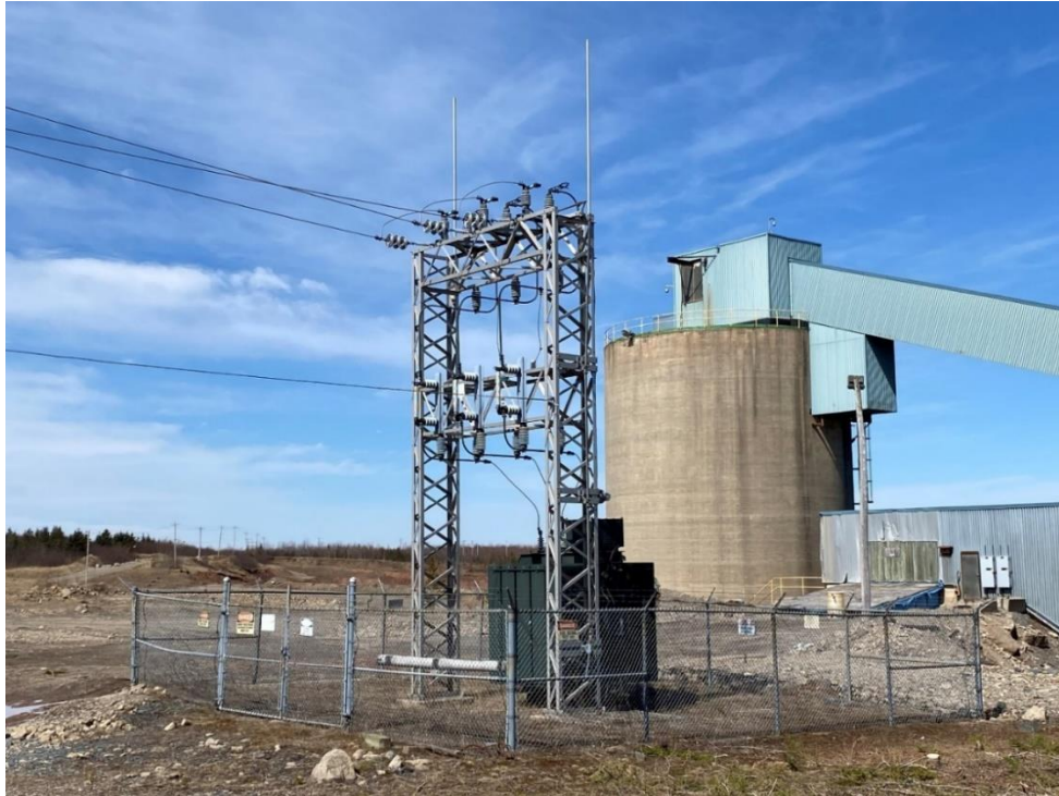
Figure 18-4: 8,000 kVA Transformer
