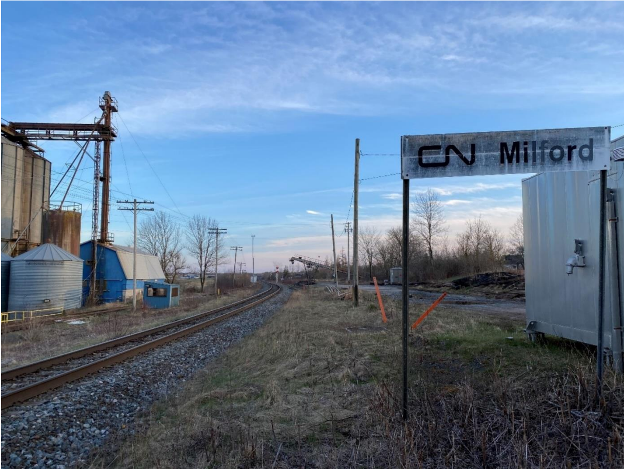
Figure 18-66: Milford CN Railway Siding
