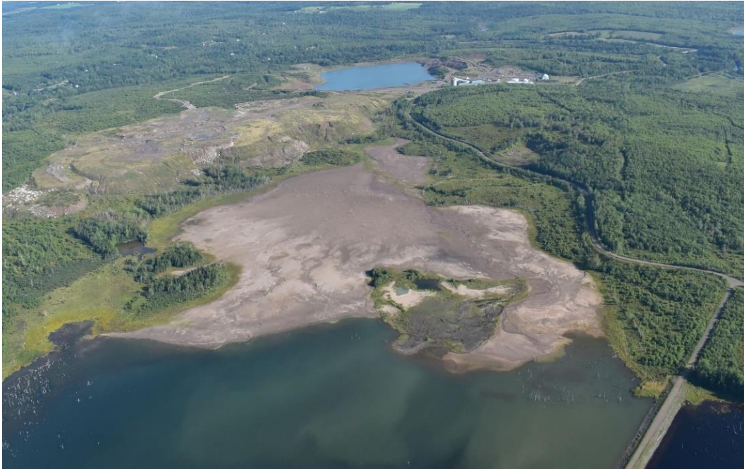
Figure 18-55: Tailings Storage Pond
