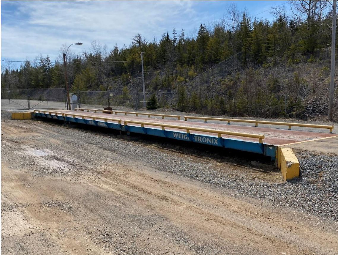
Figure 18-72: Onsite Container Weighbridge
