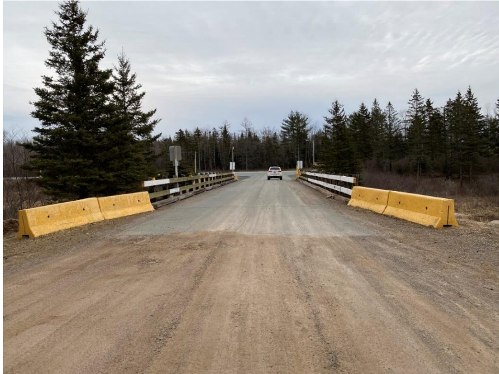
Figure 18-70: ScoZinc's Bridge & Highway Access
