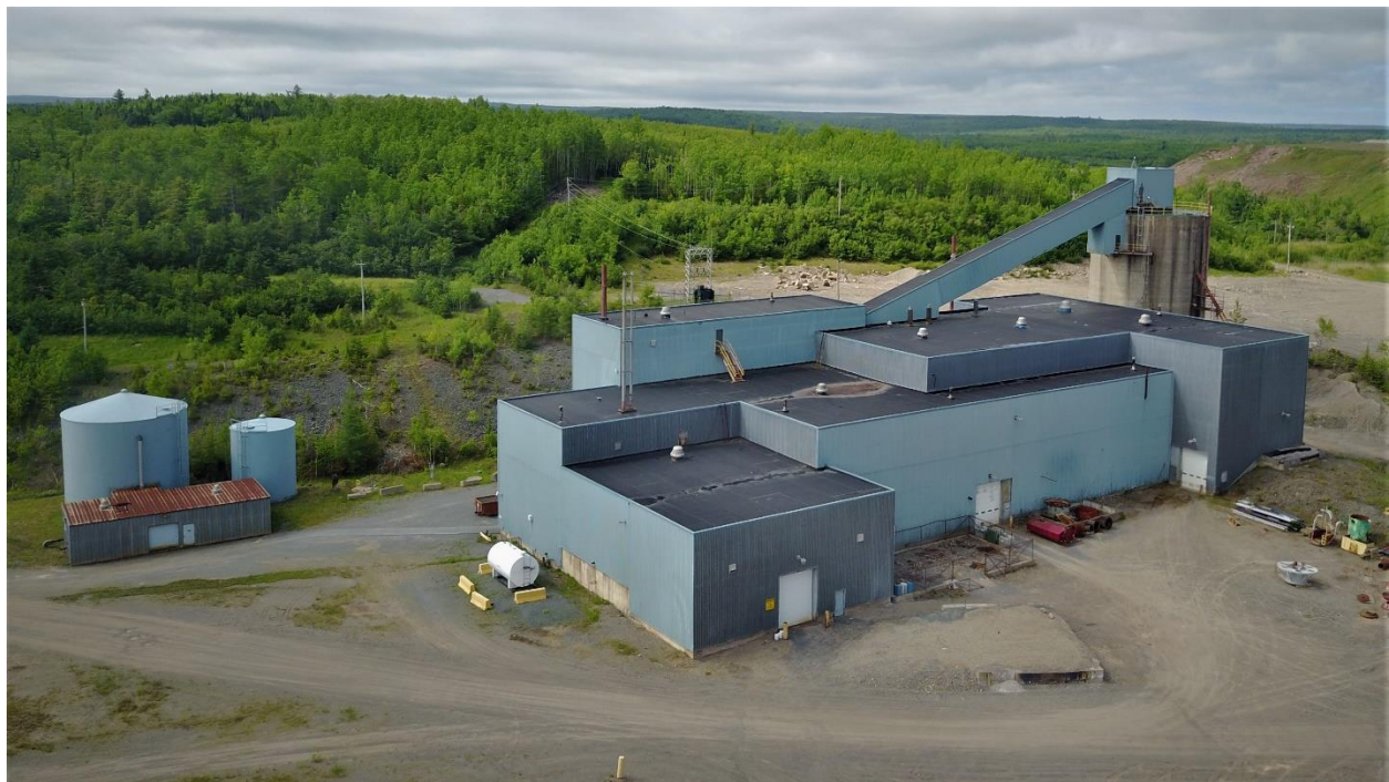
Figure 18-32: Existing Mill Processing Building – North Side Exterior View
