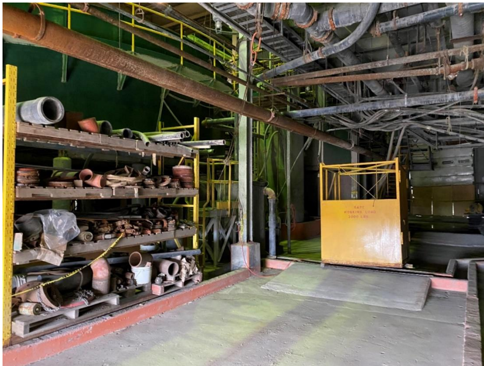
Figure 18-46: Large Ground Floor Maintenance Bays
