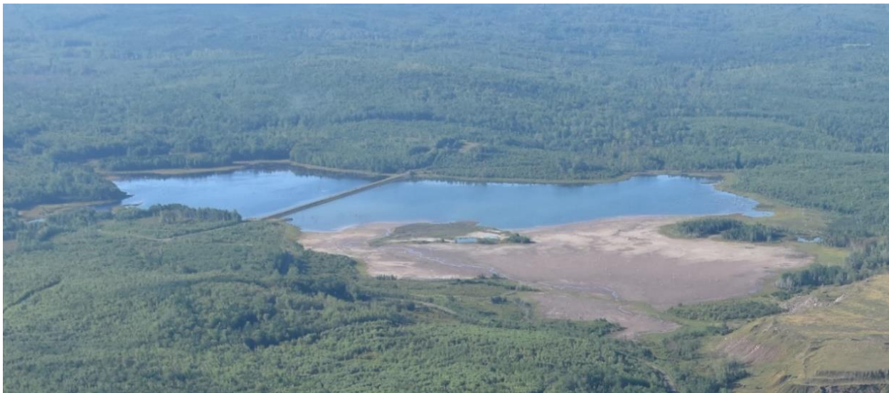
Figure 18-47: Tailings Storage Facility
