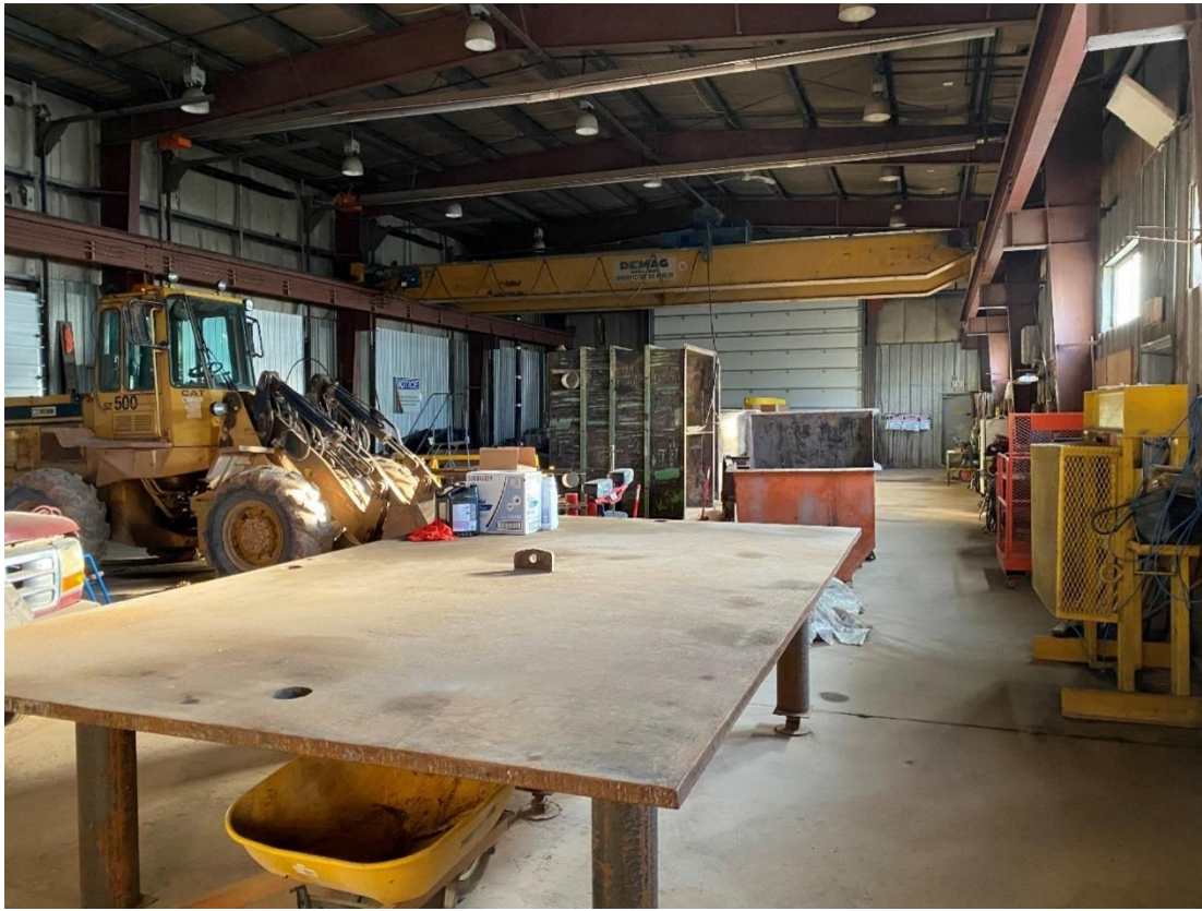
Figure 18-26: Maintenance Garage (interior)
