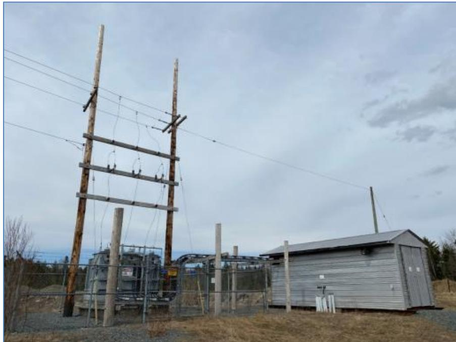
**Figure 18-5: Mine Dewatering Transformer and Substation**
