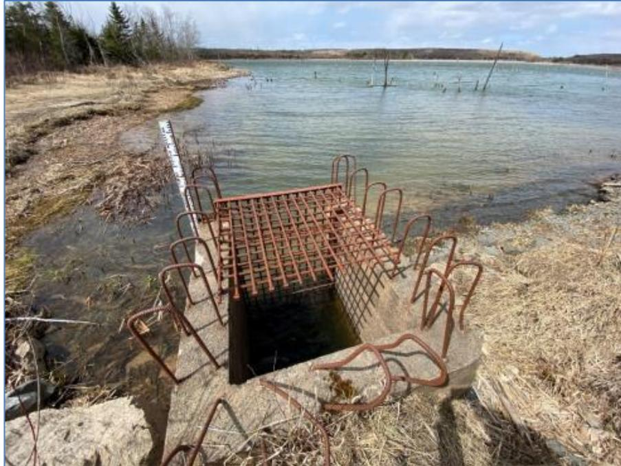
**Figure 18-48: Tailings Storage Facility Decant Tower**
