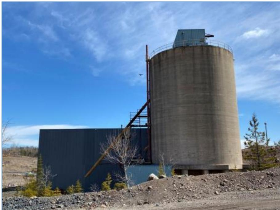
**Figure 18-33: Existing Mill Fine-Ore-Bin (Silo)**
